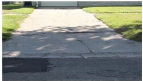
Photo 3: Cracked gutter
