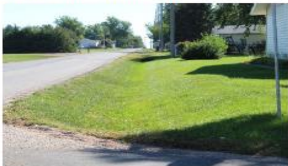
Photo 4: No curb and gutter along O Street on north and south sides
